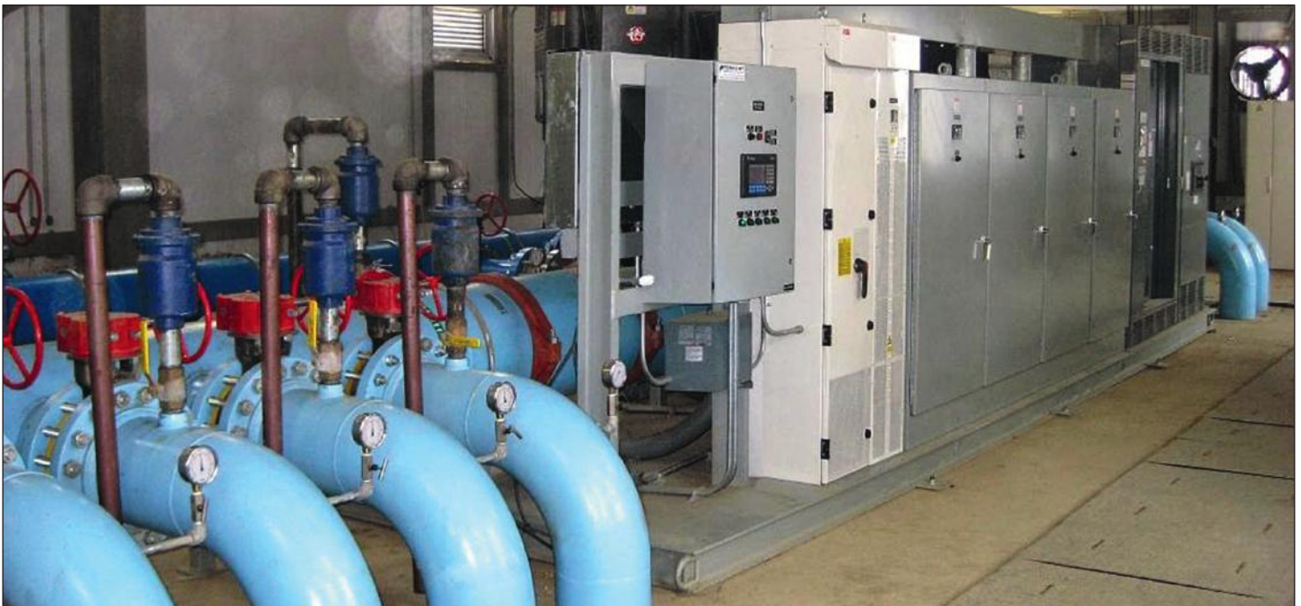
Pump station to increase pressure
