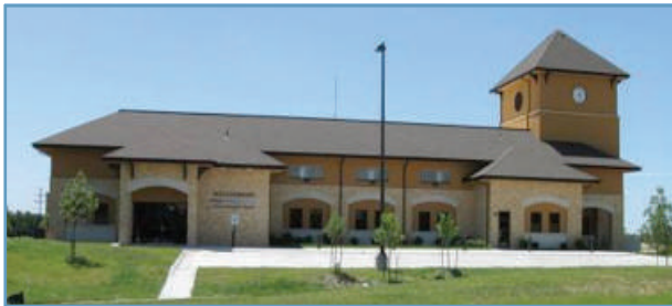
The Reverse Osmosis Water Treatment Center, Hutchinson, Kansas
