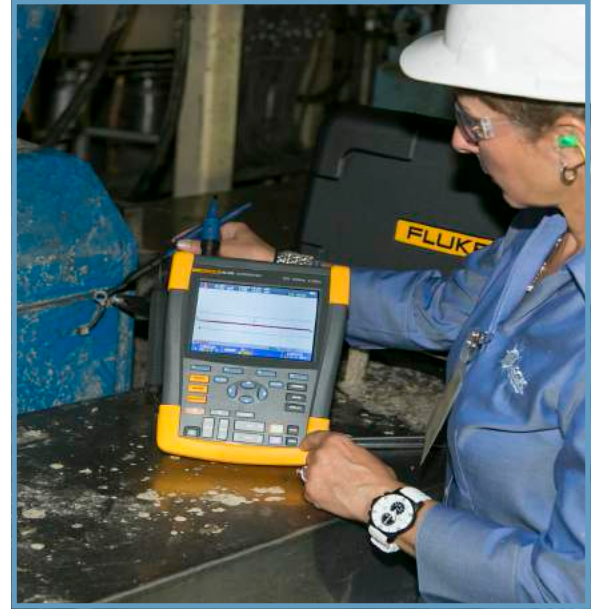
Once the AEGIS® PRO Bearing Protection Ring had been installed and the motor restarted, an AEGIS® technician confirmed that motor shaft voltages were minimal using an oscilloscope. A special "pigtail" lead allows maintenance personnel to periodically check the voltages (and therefore the likely condition of the bearings) safely and easily, without exposing the shaft. The ring has been diverting potentially damaging voltages to ground since it was installed.
